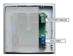
The RJ11 jack marked for telephony (at the right of the NTP) can only be used when a telephony cable is installed between the modem (VoIP output) and the green terminals of the NTP.
